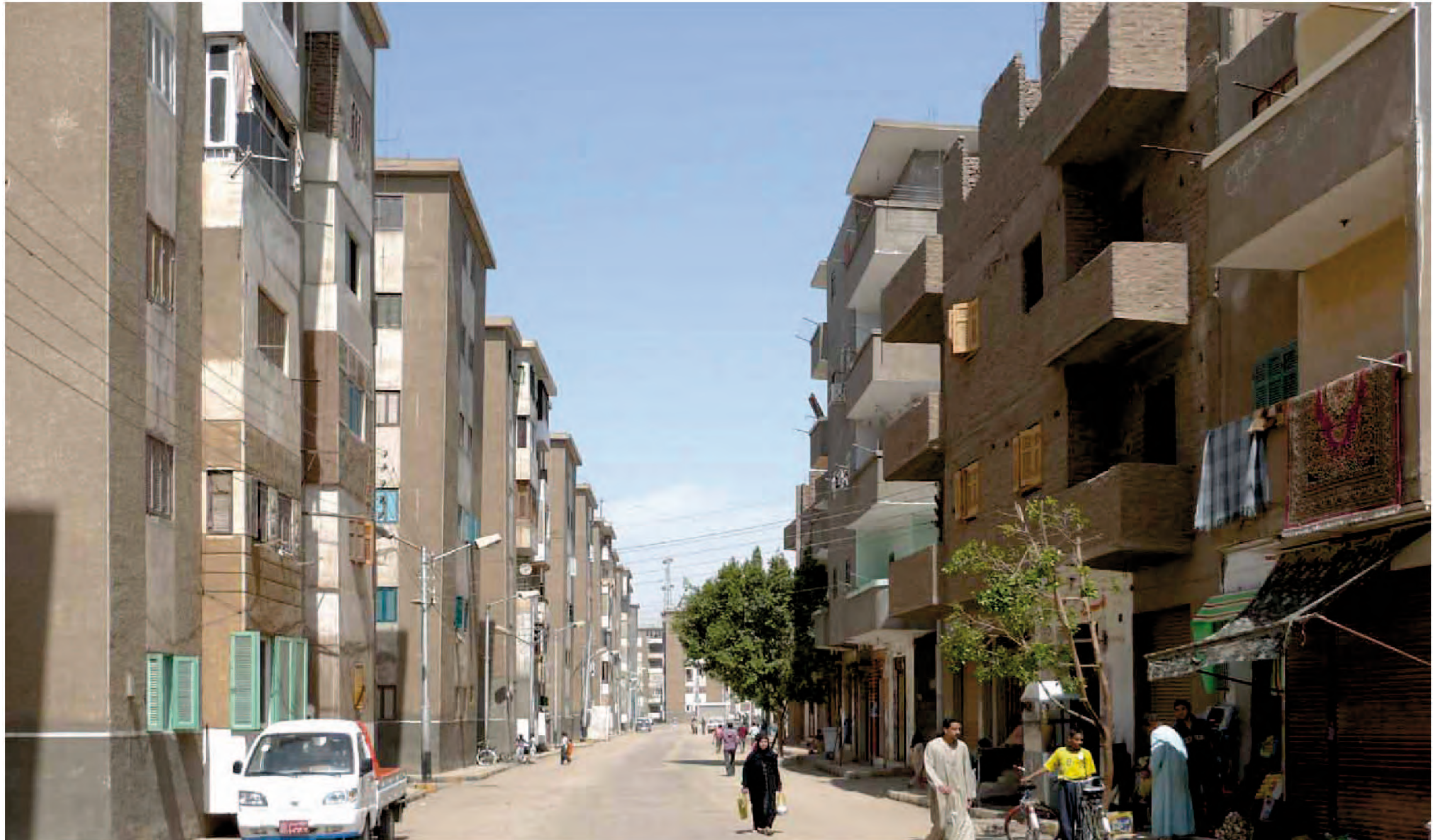
Decaying Public Housing
