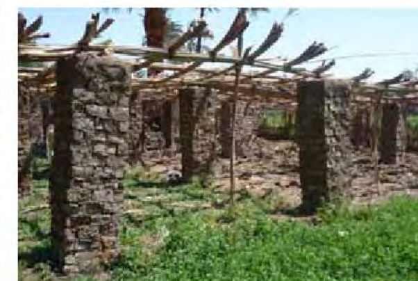
The construction for grapes, which consists of stone pillars and palm leaves, is built by the farmer.
